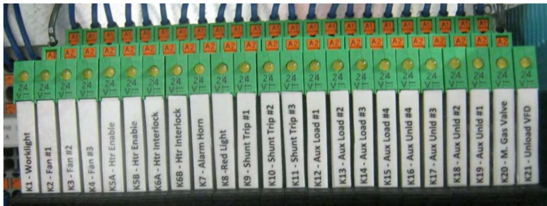
K relays energized by 24VDC from PLC
