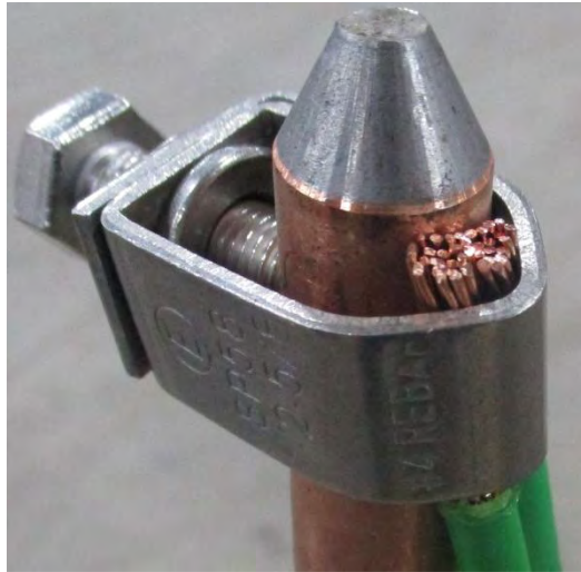
Wires clamped to ground rod
