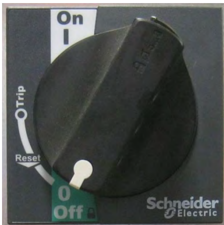
Image 2 – Main Disconnect switch
