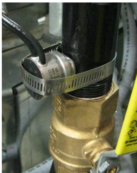
Image 4-4 – Vapor over-temp switch
