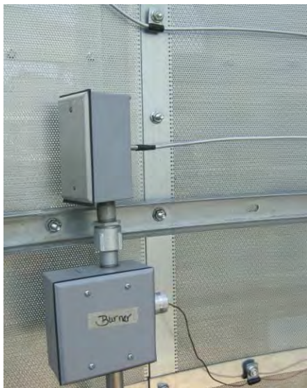
Image 24 – Plenum RTD, capillary box
