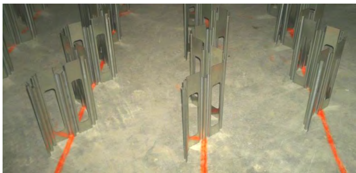
Image 3 – Positioning SuperWave Supports
