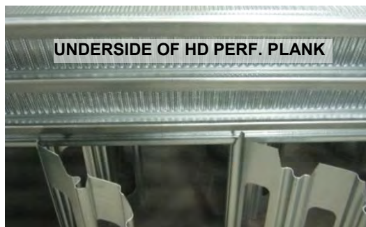
Images 5 & 6 – Positioning Heavy-Duty Perforated floor plank on SuperWave Supports
