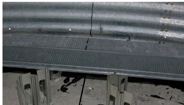
Image 3 – Marking bin wall, installing first plank
